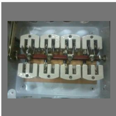
Electrical Switchgear & change over switch
